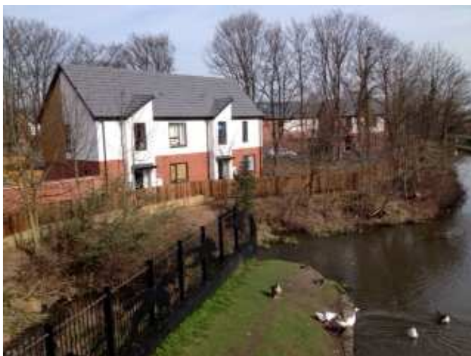
Stanyon's Yard, Dallow Bridge
