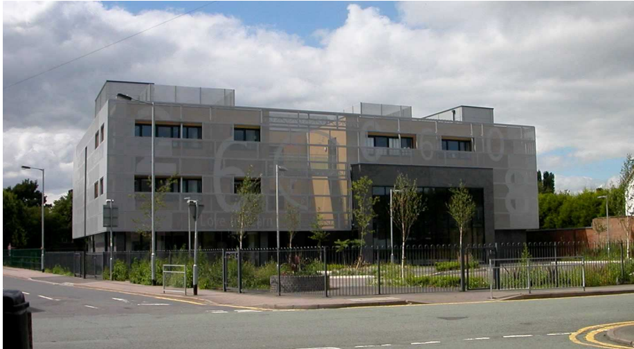
Christ Church Primary School, Uxbridge Street
